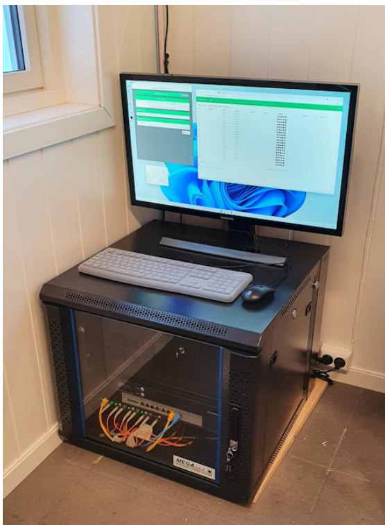
Example of rack with USP, Server and fiber adapter. WiFi antenna outdoor.
